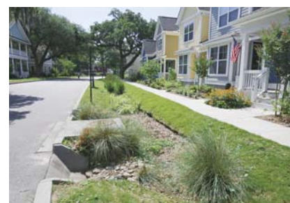
Planned green areas constructed throughout a city can absorb rainwater and help reduce flood damage and improve water quality.
